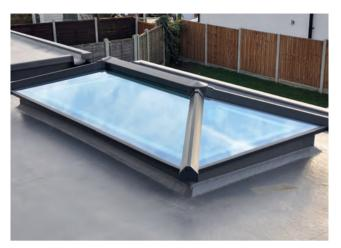
▲ Figure 3.14 Natural light entering a building through roof lanterns
