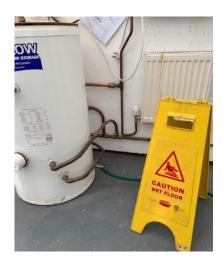
Preparation for draining down: correct equipment and drain point used to drain down system pipework for decommissioning activities.
