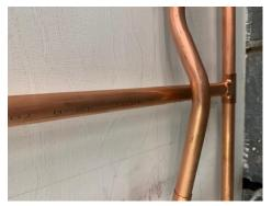
Fabricated passover with appropriate clearance. no signs of throating or rippling.
