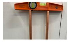
Pipework level and within tolerance. (+/-2mm)
