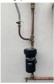
Component fitted correctly with no signs of tool marks from installation.
