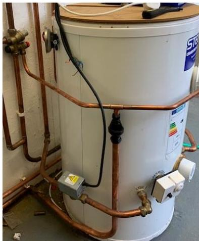
Pipework installed to the required tolerance ( $\pm 2\text{mm}$ ). Bends have been completed to a high standard with no signs of throating or rippling.
