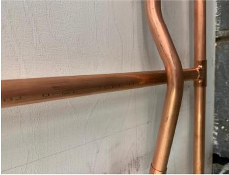
Fabricated passover with appropriate clearance. no signs of throating or rippling.
