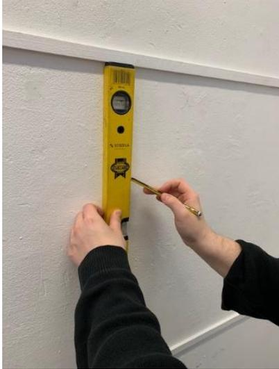
Candidate marking out a work area using a spirit level to provide a straight and vertical line on the first attempt.
