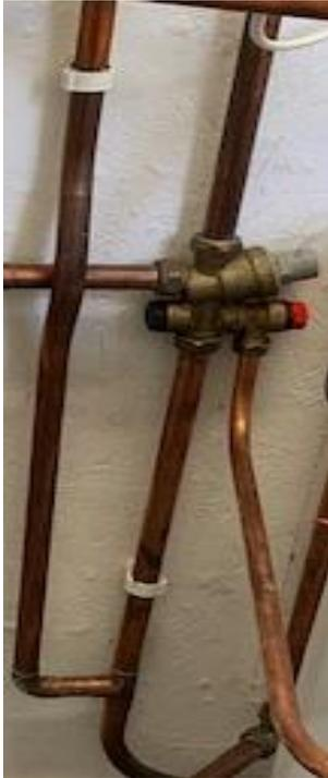
Pipework level and adequately clipped with appropriate spacing. Pipework fabricated without the use of additional fittings.
