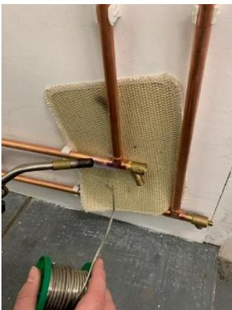
Correct use of blow lamp, safe soldering, correct selection of solder, protection of customer property with heat mat centrally positioned. Removal of vulnerable heat sensitive components before soldering commences.
