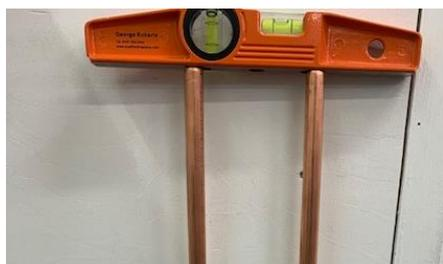
Pipework level and within tolerance. ( $\pm 2\text{mm}$ )
