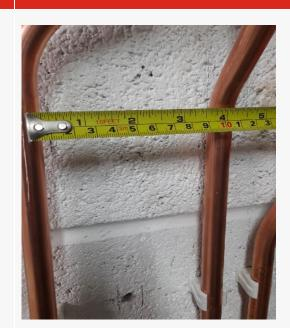
Tolerances (+/-5mm) have been met during the installation of pipework.
