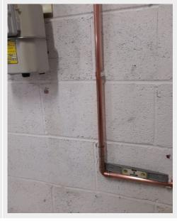
Components correctly installed but not level.
