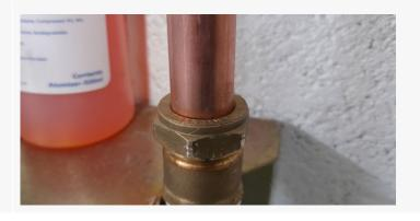
Soldering/soldered fittings to show that heat mats have been used and no burn/scorch marks to the wall/or burn marks to the wall to support the assessors making of the jointing process.
