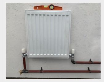
Finished installation and associated pipework including the installation of both functional and safety controls.
