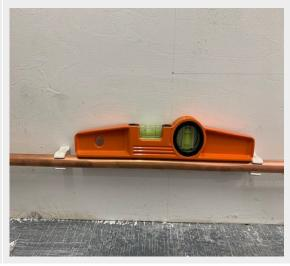
Components correctly installed but not level
