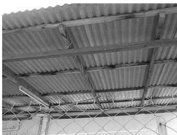
Figure 2 Asbestos roof of the football stand to be demolished
