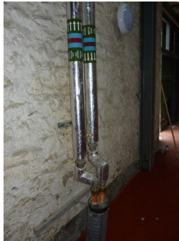
DH pipework route from boiler house
