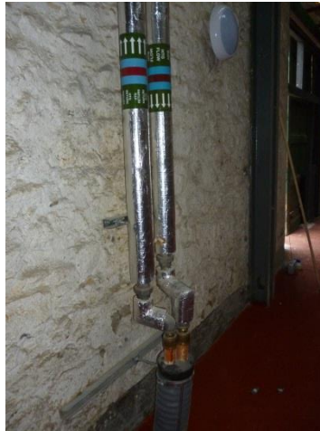
DH pipework route from boiler house
