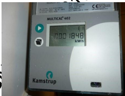
Each property is metered for hot water demand
