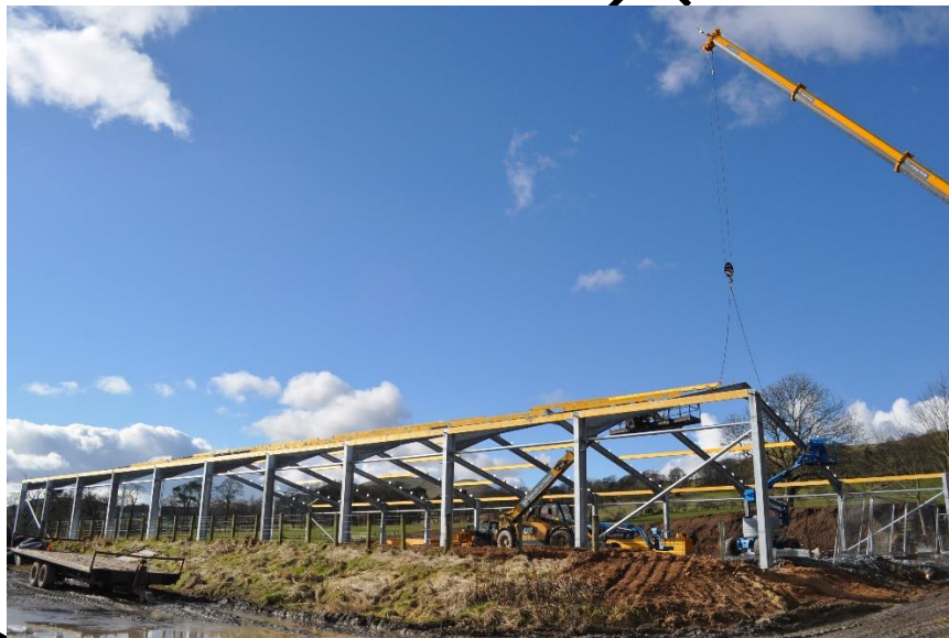
Steel portal frame construction progress
