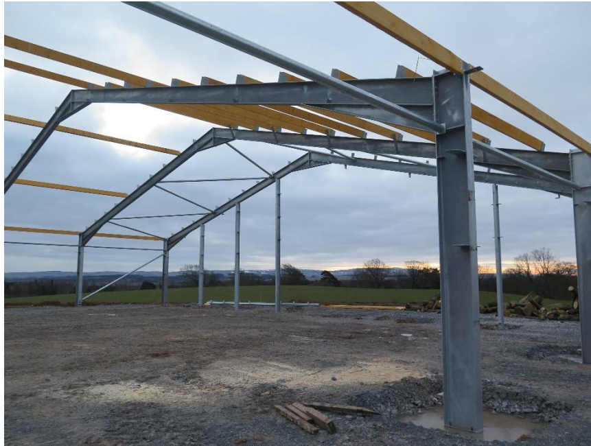
Steel portal frame construction progress
