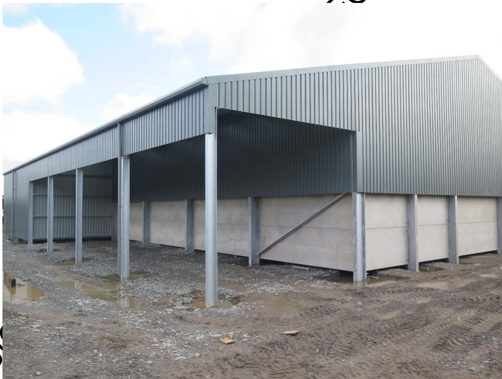
Steel portal frame construction near completion
