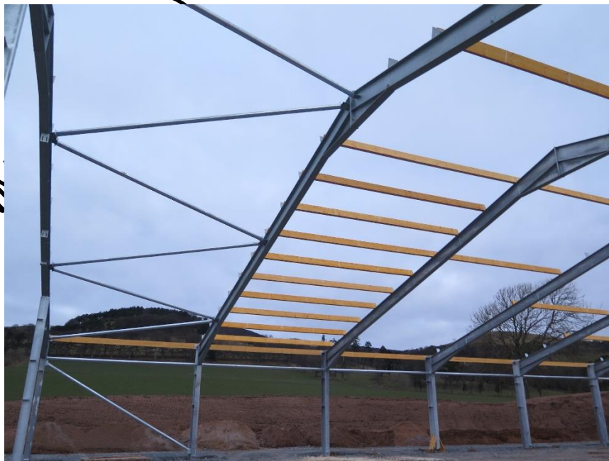
Steel portal frame construction progress
