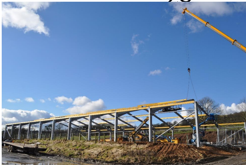
Steel portal frame construction progress
