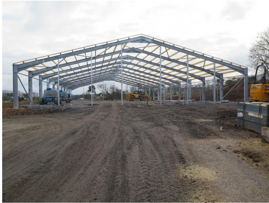
Steel portal frame construction progress
