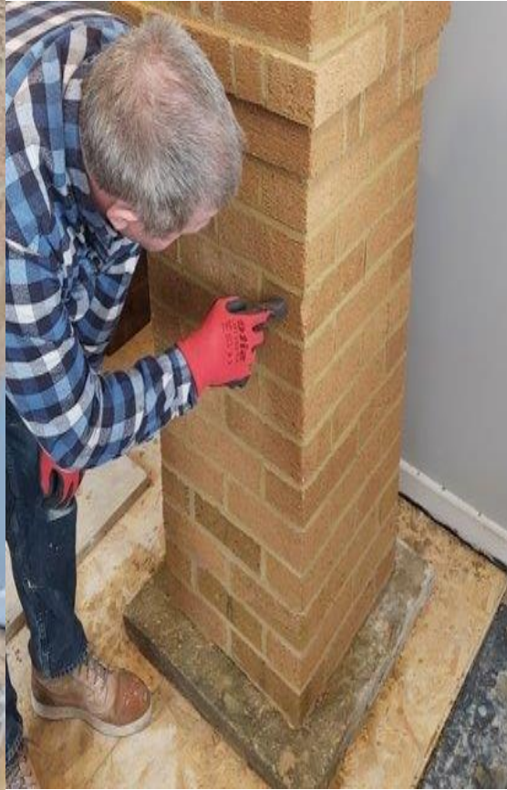
Photograph 32 showing removal of materials for preparation or repair (chipped brick)
