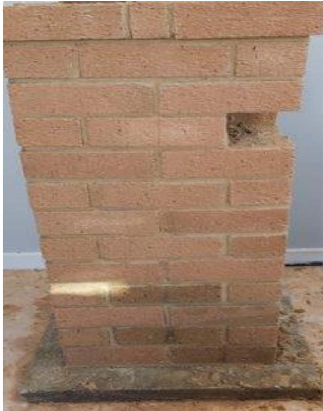
Photograph 32 showing removal of materials for preparation or repair (chipped brick)
