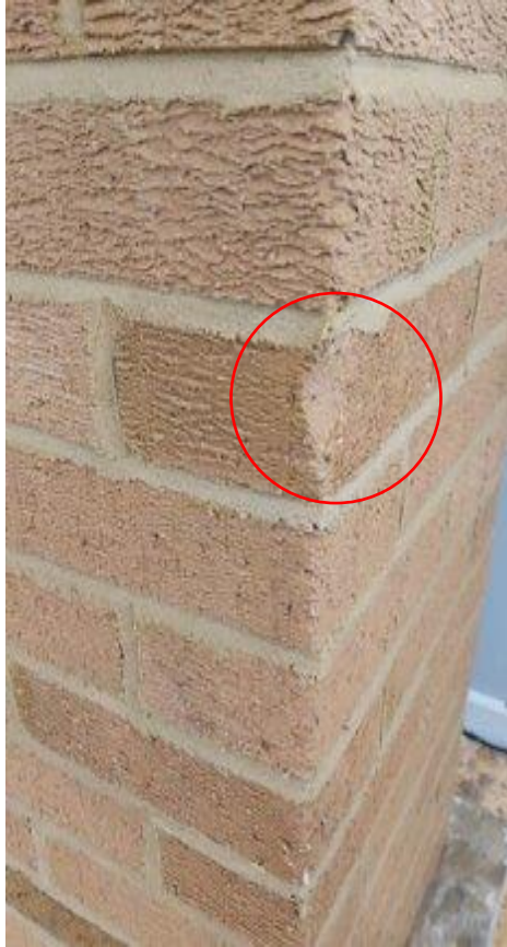
Photograph 32 showing removal of materials for preparation or repair (chipped brick)
