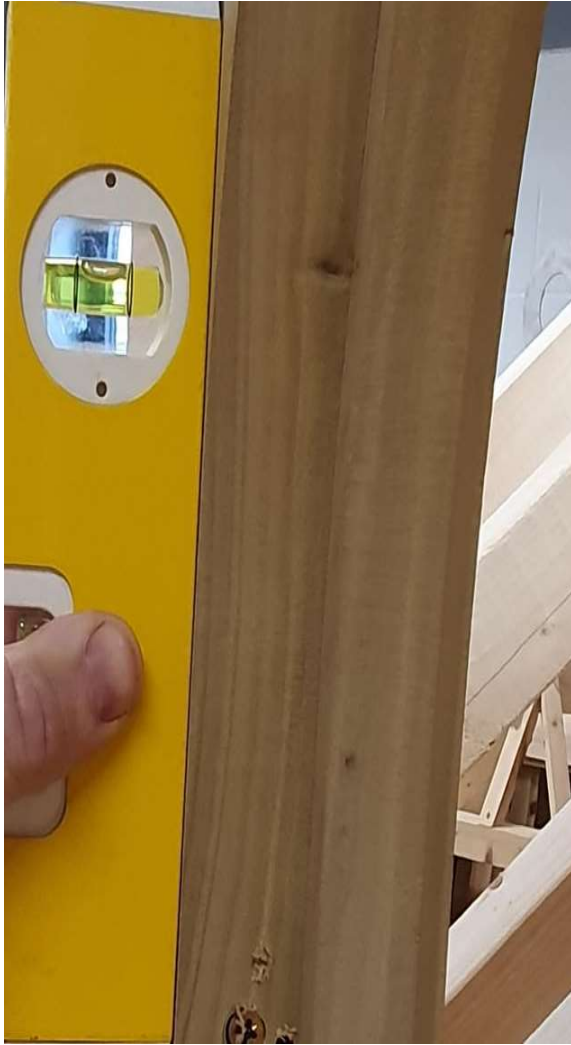
Gothic window installed plumb to the dormer within 0.5mm.
