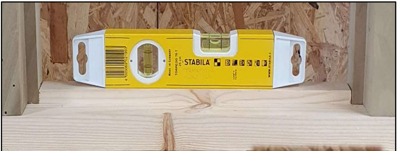
Photographs 19 – 23 – Images show plumb spaces and level of window fitting, with the window installed level in the dormer within 0.5mm.
