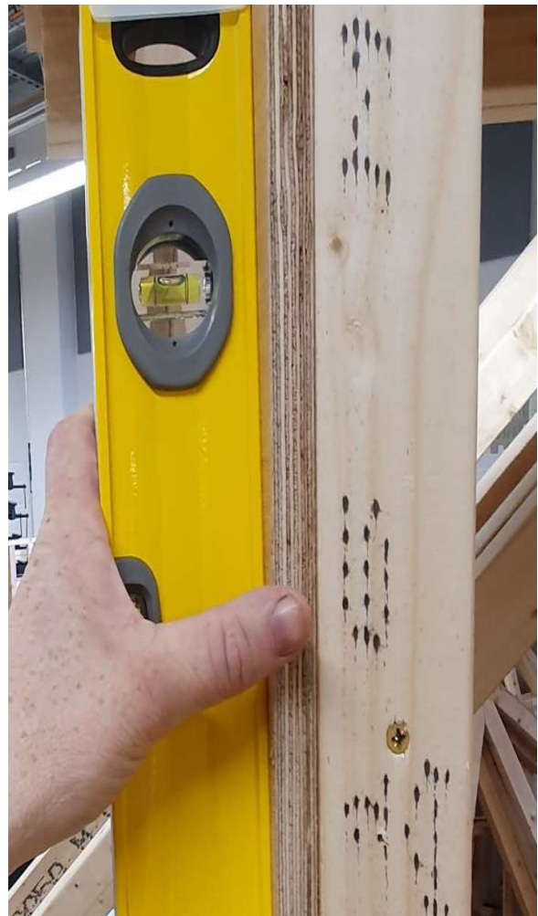
Dormer face plumb within 1mm.
