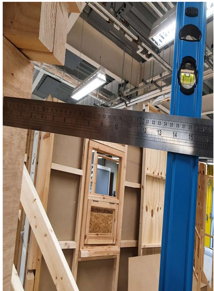
Dormer face within 5mm of the stated 400mm.
