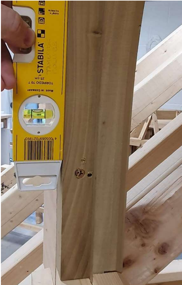
Gothic window installed plumb to the dormer 2mm out of plumb, but within tolerance.
