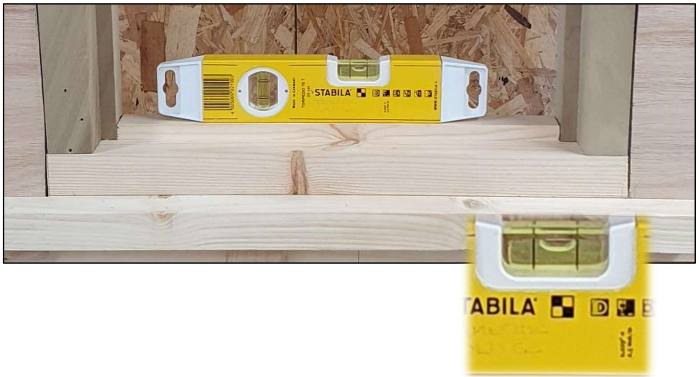
Photographs 20 - 24 – Images show plumb spaces and level of window fitting, with the window installed in the dormer 2mm out of level but within tolerance.
