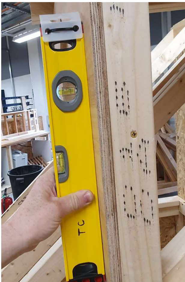
Dormer face plumb within 3mm.
