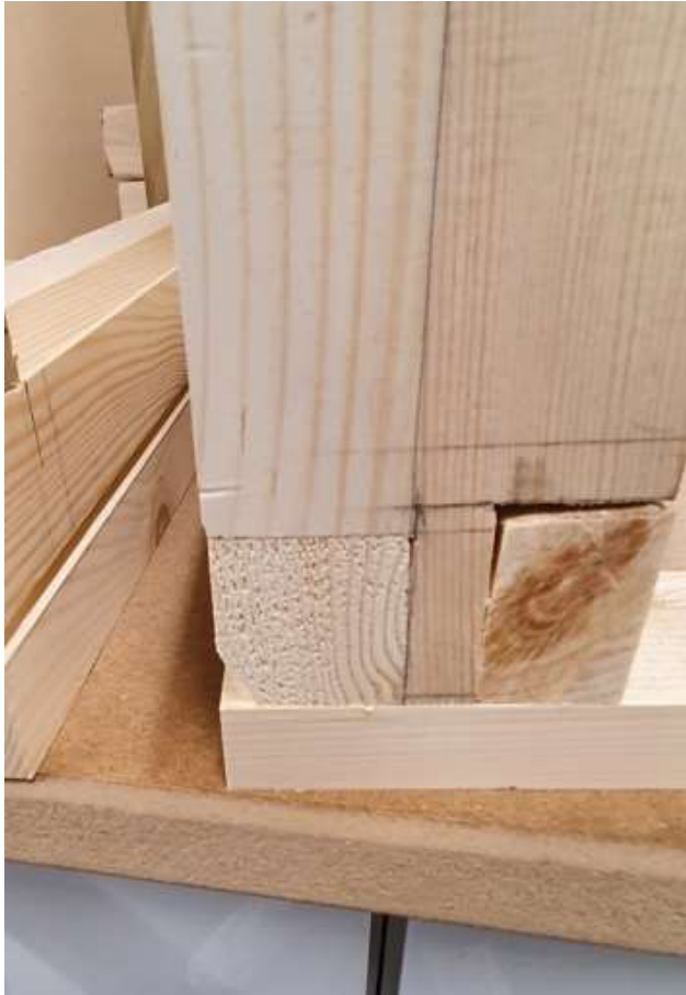
Photograph 19 – Image shows close up of horns cut off and finish to the ends, rebated mortise and tenon with slight gaps not exceeding 3mm.
