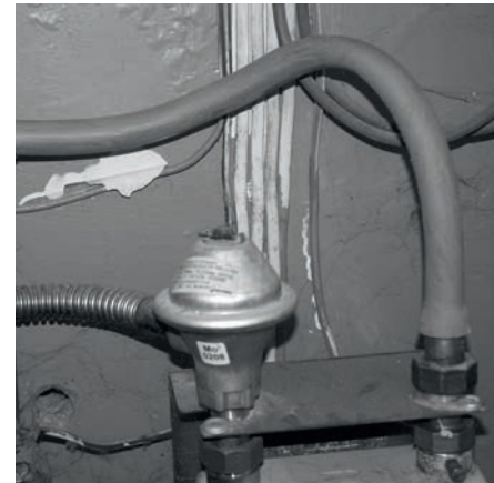
Lead pipe on the outlet of a meter
