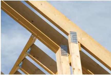
Roof trusses are made with butt joints fixed with nail plates
