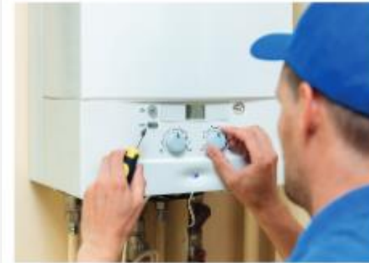
▲ Figure 3.17 Retrofit installer fitting an energy-efficient boiler
