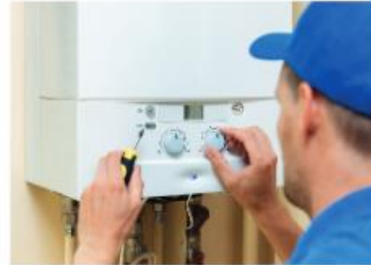
▲ Figure 3.17 Retrofit installer fitting an energy-efficient boiler
