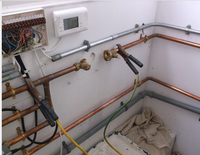
Task 3 Photo ref 4. Circulator removed after isolation at valves.
