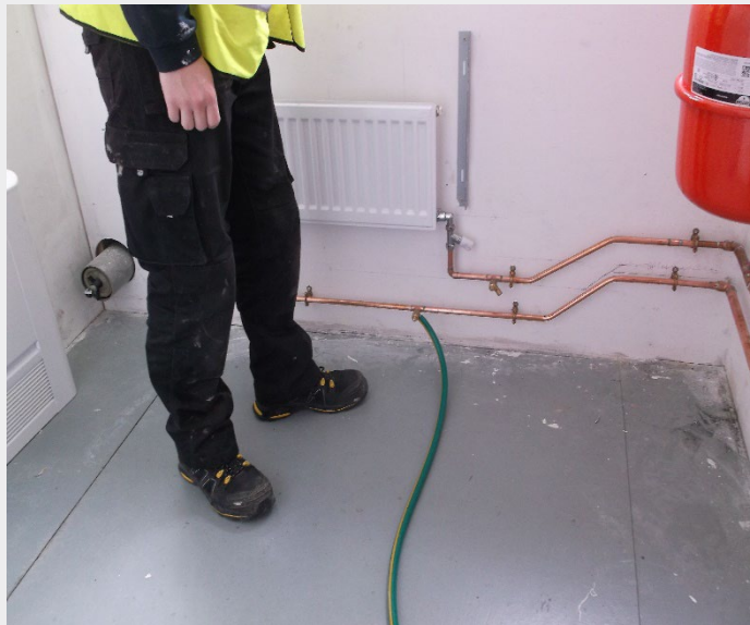
Task 2 Photo ref 17. Draining system with hose pipe to lowest drain in floor gully Hose was run across floor safely with Aboard signage
