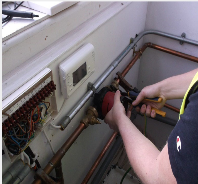
Task 3 Photo ref 5. Circulator installed with correct direction of flow. The valves were opened, and joints visually checked for leaks, <first name> checked the system pressure gauge and was happy the gauge read 1 bar.
