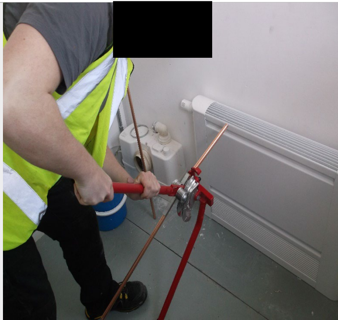
Task 2 Photo ref 7. <first name> fabricating the 15mm Offset bend for LST radiator flow pipe.
