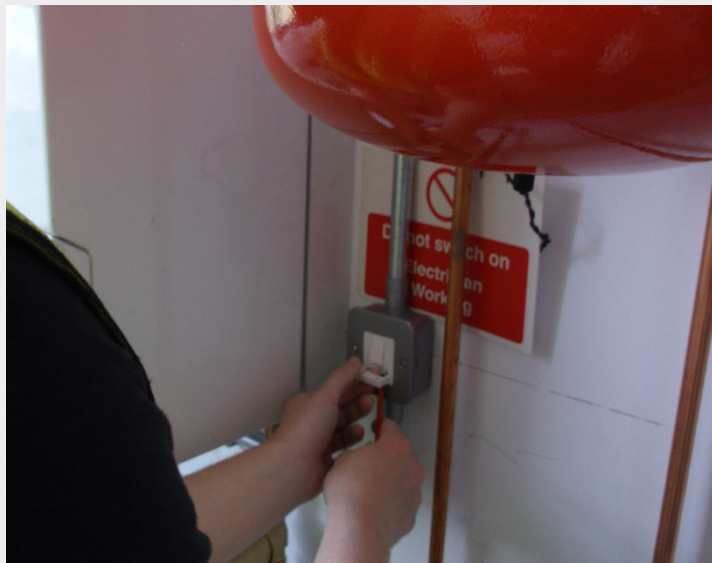
Task 3 Photo ref 3. Safe isolation of the heating system. Fuse removed and warning sign above switched fuse spur.
