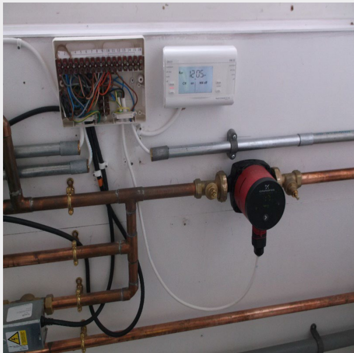
Task 3 Photo ref 7. Circulator installed, new cable and plug wired to the wiring centre and electrical supply restored.
