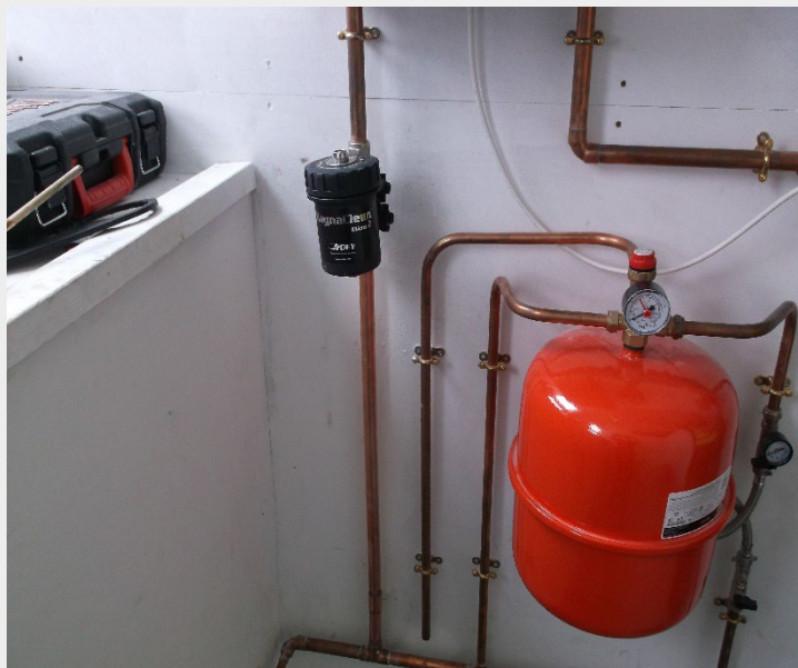
Task 2 Photo ref 2. Magnetic filter installed without any clips.
