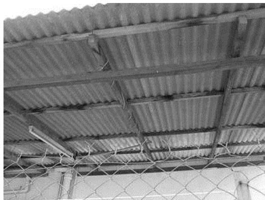
Figure 2 Asbestos roof of the football stand to be demolished
