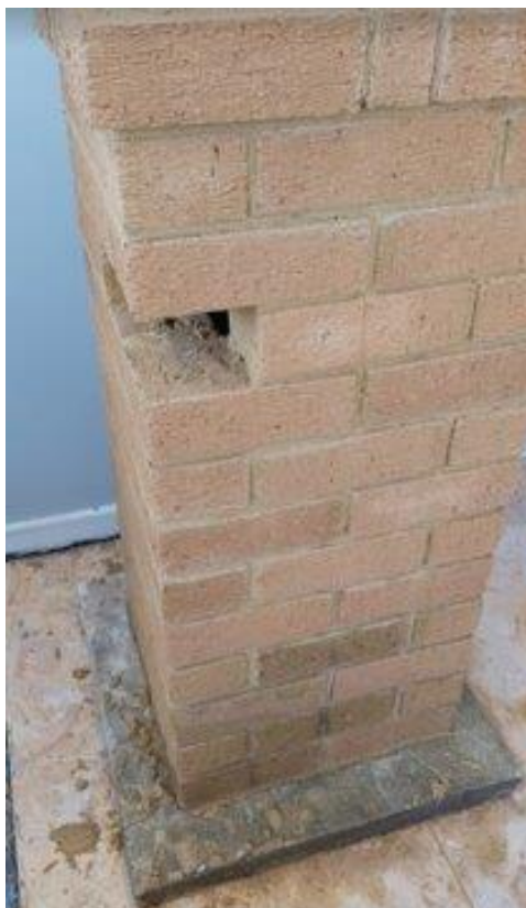
Photograph 39 Removal of mortar
