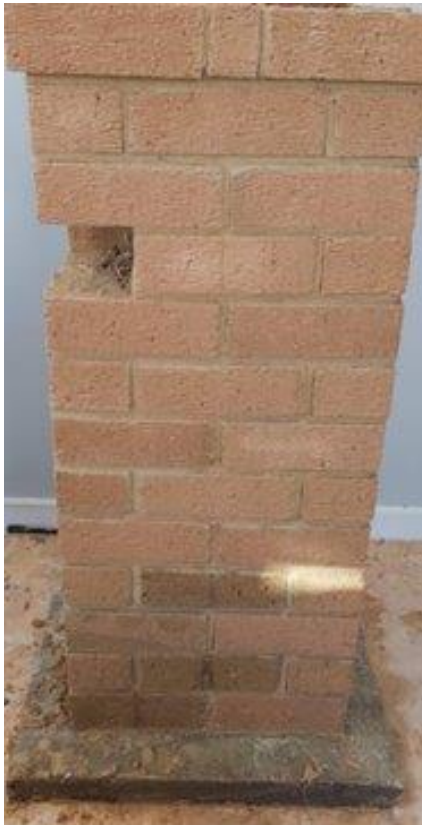
Photograph 38 Removal of brick
