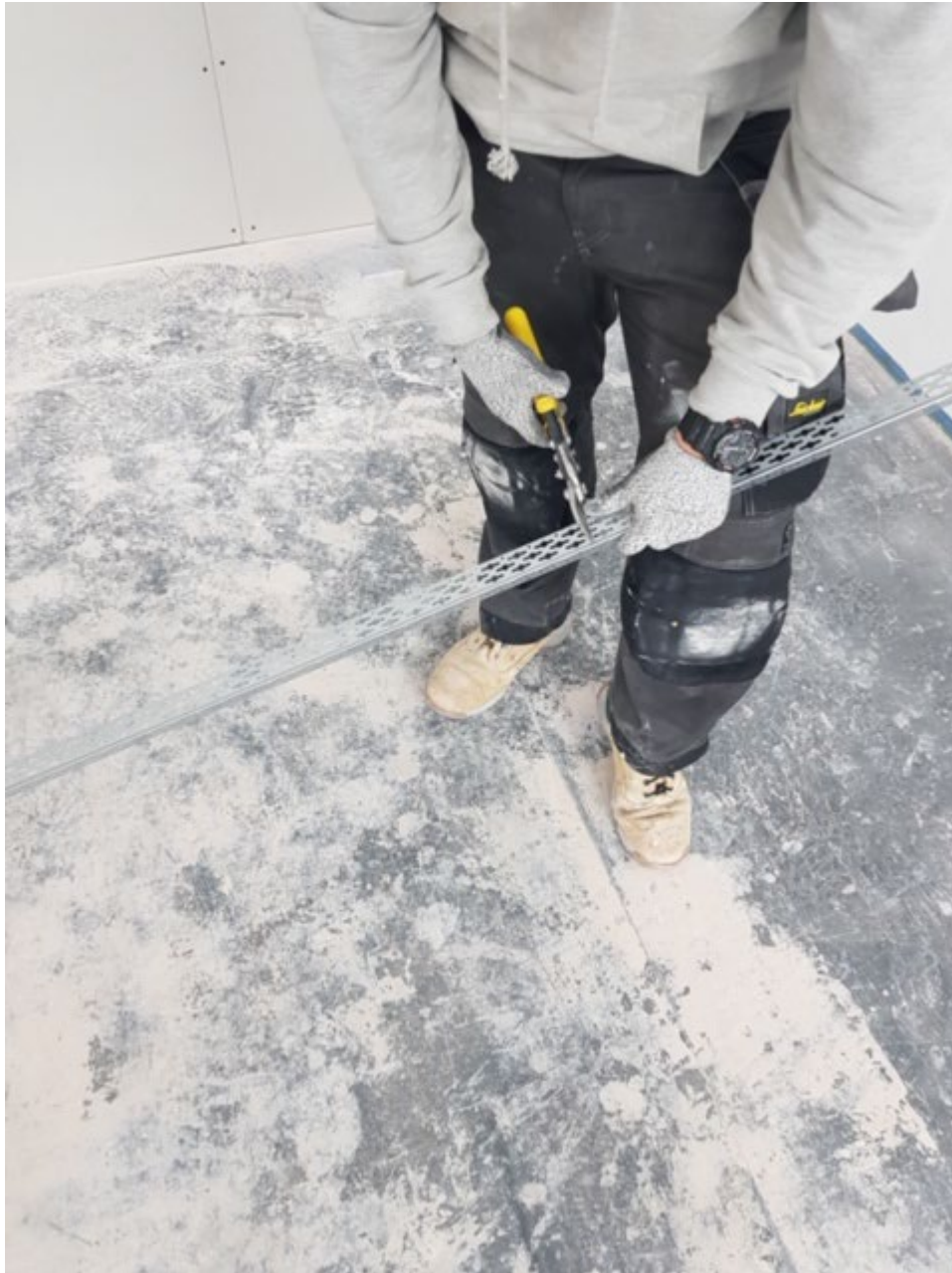
Photograph 18: Showing techniques used to cut (from taken dimensions) thin coat angle beads (prior to positioning)
