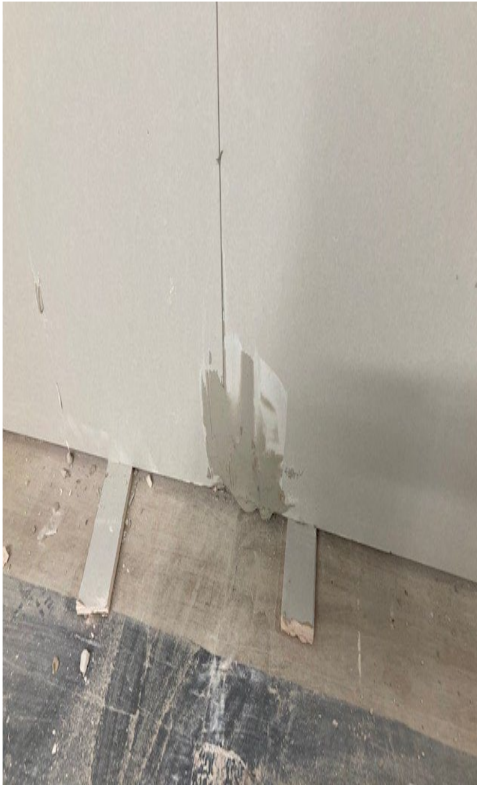
Photograph 16: Showing rectification/filling in of damaged plasterboard following positioning
