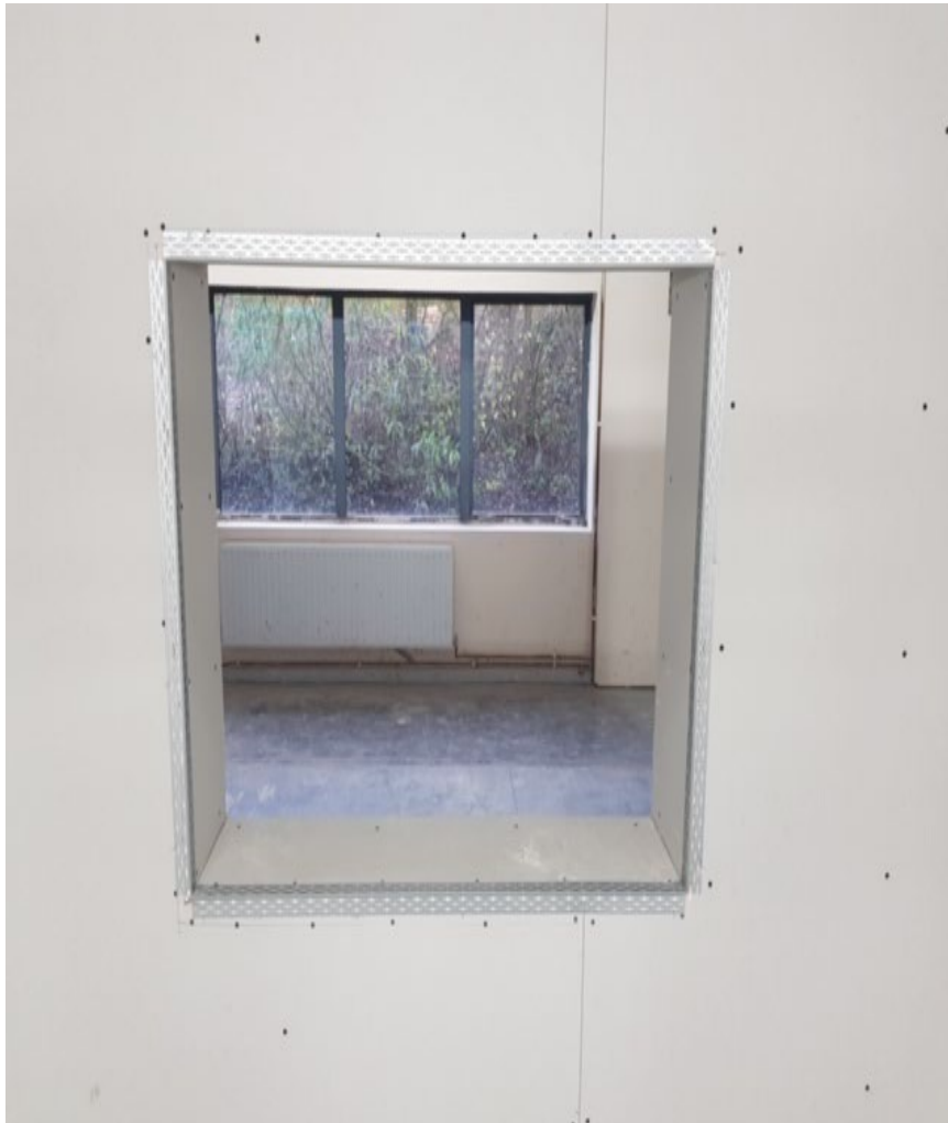
Photograph 22: Completed thin coat beads
