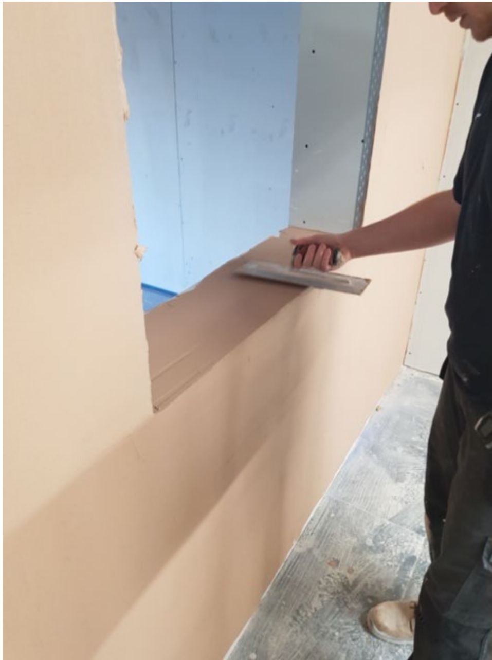
Photograph 27 – Showing plaster application in production
