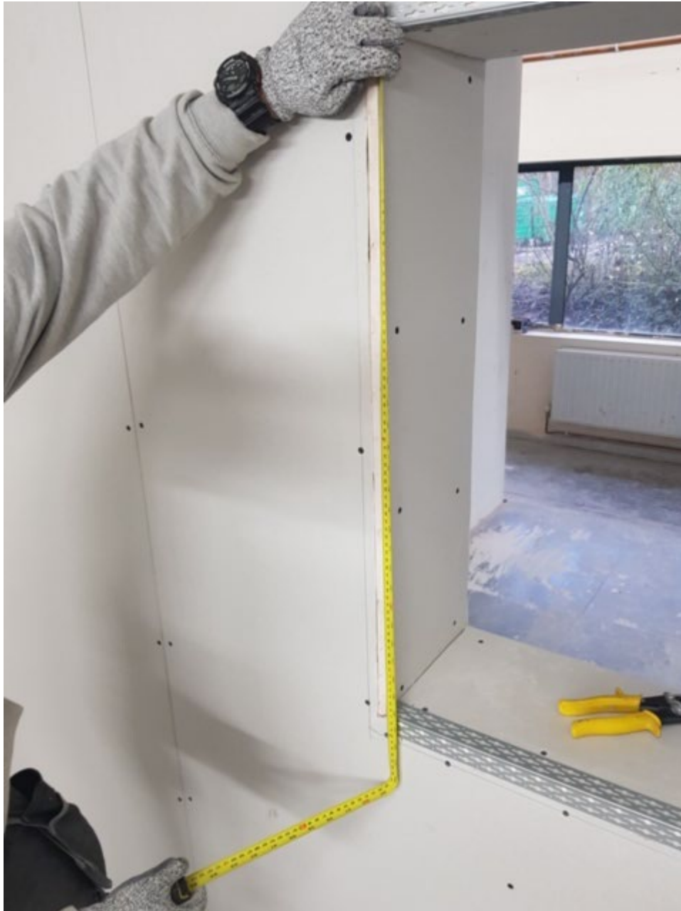
Photograph 20: Showing measurements retaken to rectify cutting/measurement error on one window return
