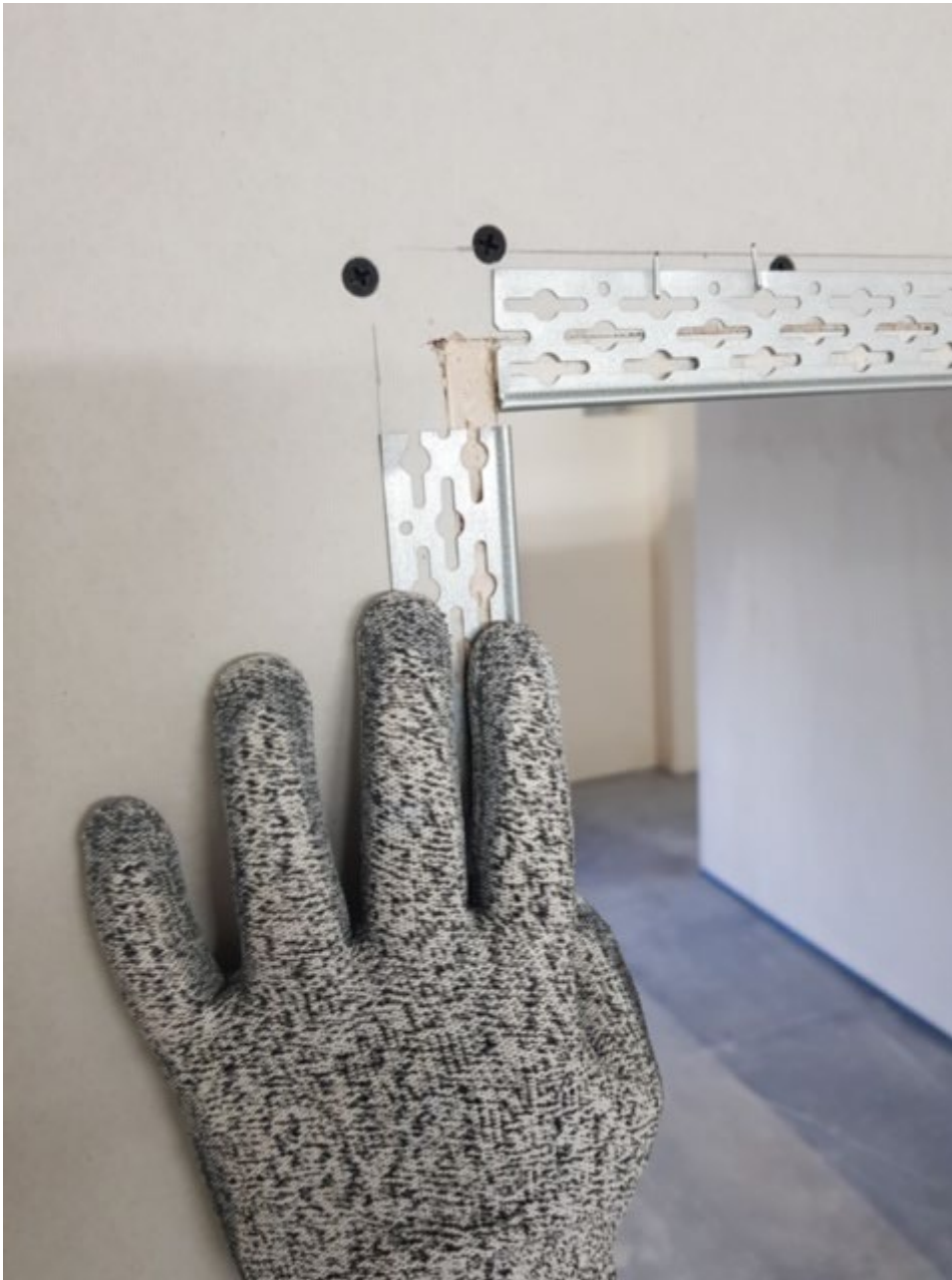
Photograph 19: Showing positioning of beads
