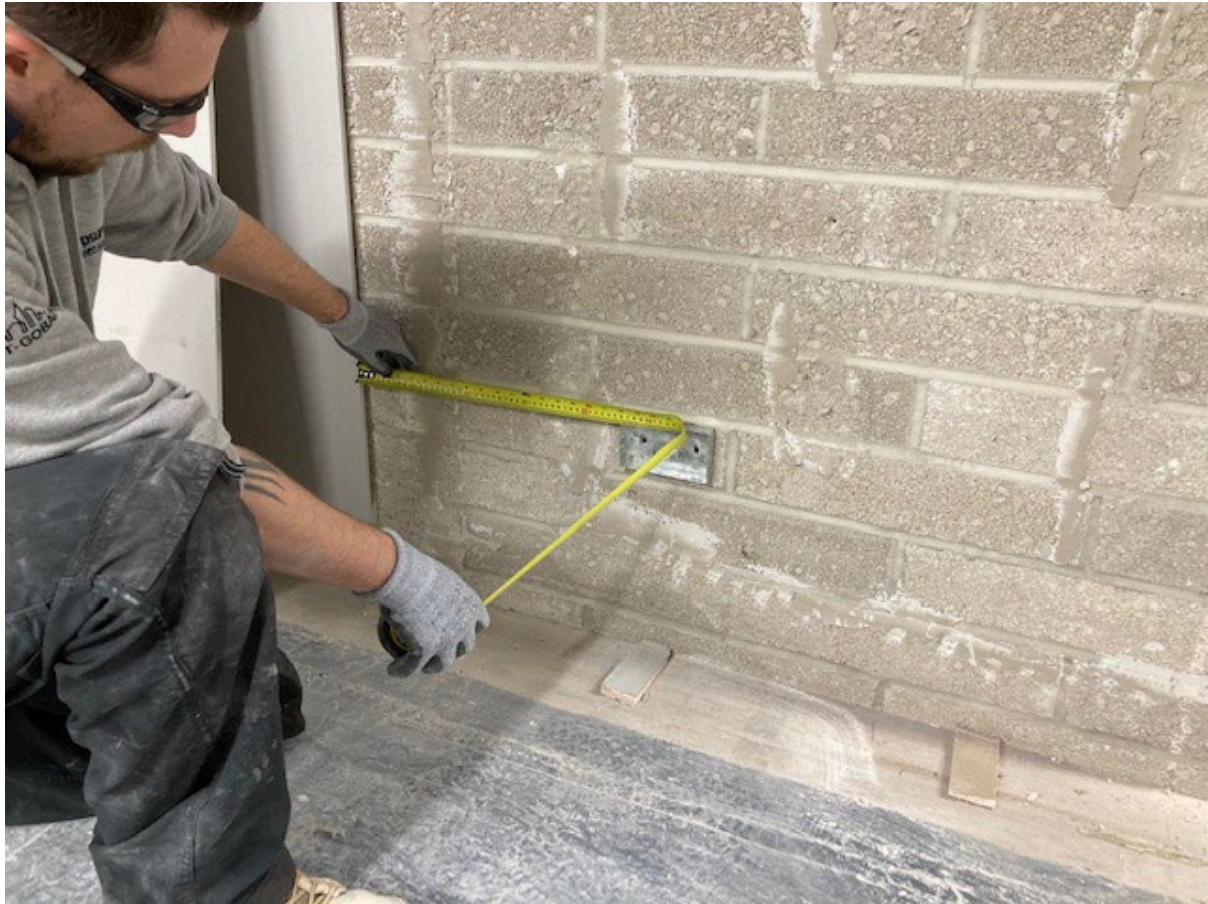
Photograph 2 – Showing accurate measurements for service box for transfer to plasterboard
