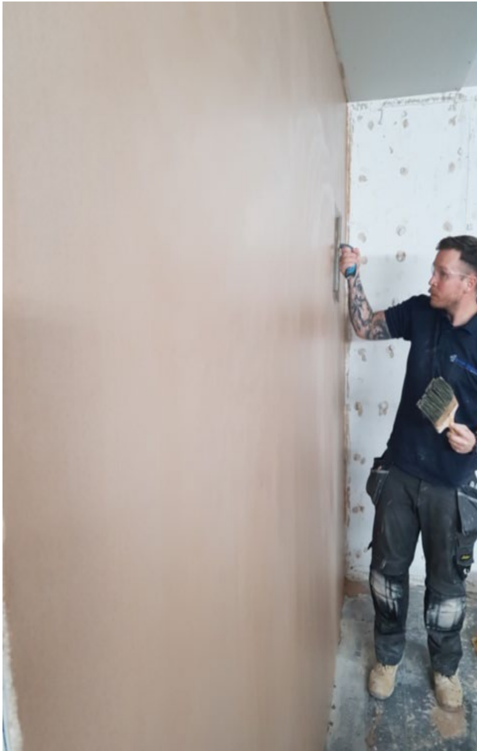
Photograph 28 – Showing completion of plaster finish
