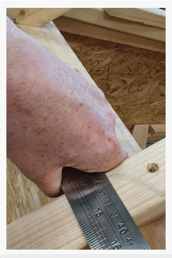
Rafter plumb fascia cut not within 3mm to the stated 150mm overhang, (142 mm).
