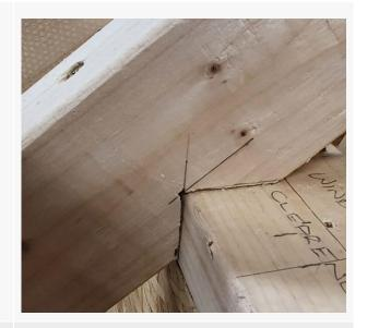
Rafter plumb cut tight to wall plate with no gap exceeding 1mm. Securely fixed.
