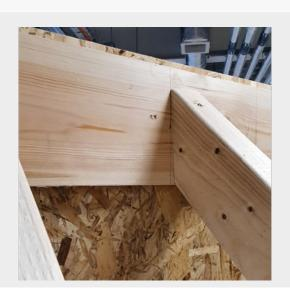
Rafter overhang run in line with gaps not exceeding 1mm.
