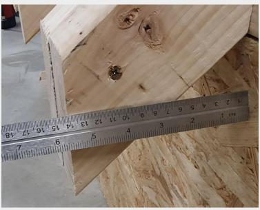
Gothic window installed plumb to the dormer 2mm out of plumb, but within tolerance.
