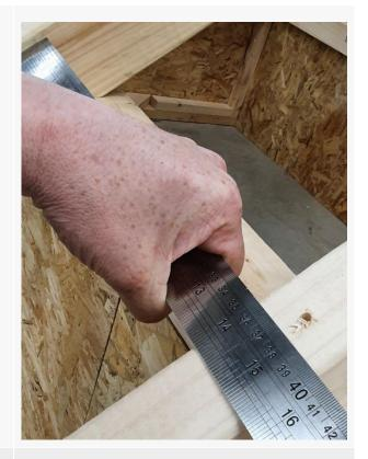
Rafter plumb fascia cut within 1mm to the stated 150mm overhang.
