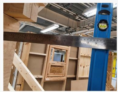
Rafter plumb cut with a gap within 3mm tolerance. Securely fixed.
