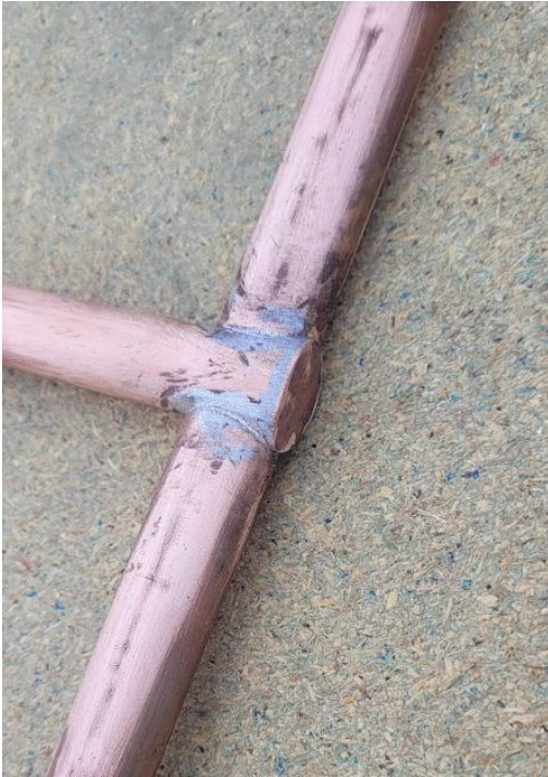
Photographs 8 and 9 show attention to detail, with the joints and lightning cable soldered into position.
