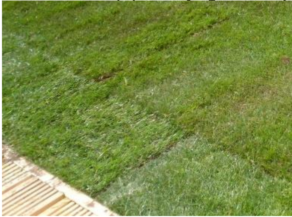
Photo evidence (iv) Turf laying: Photo of joints after butting up.
