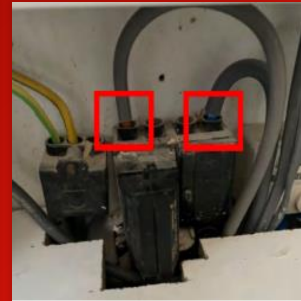
Meter tails double insulation not taken into enclosure (ID186)
