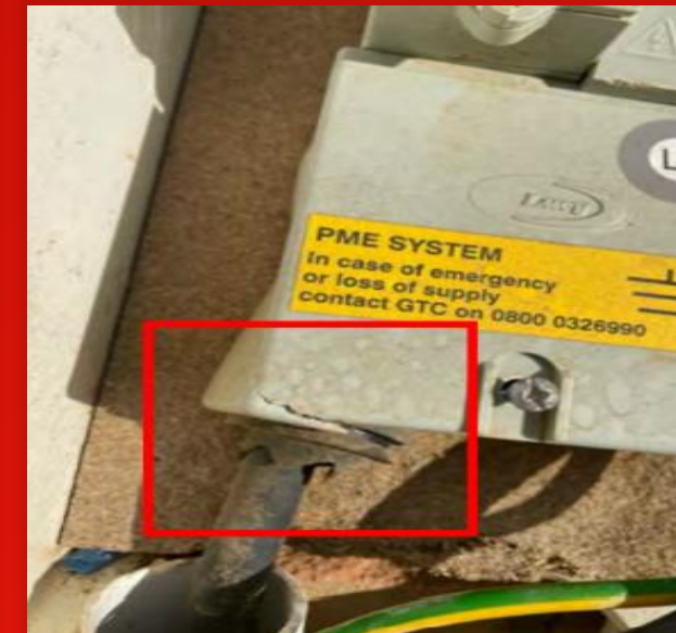
Seal ring of fuse carrier broken (ID706)
