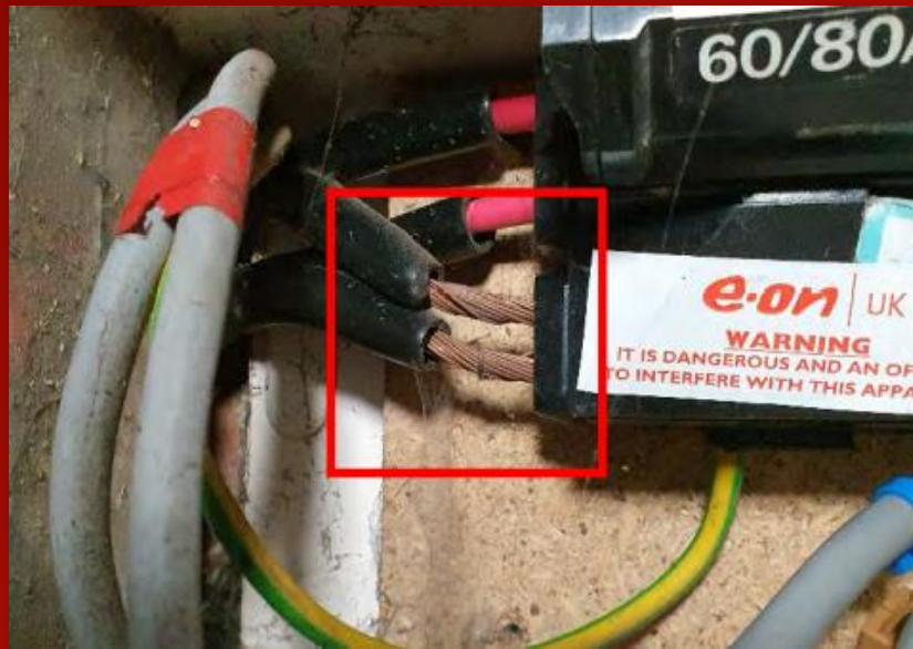
No insulation on service head (ID466)
