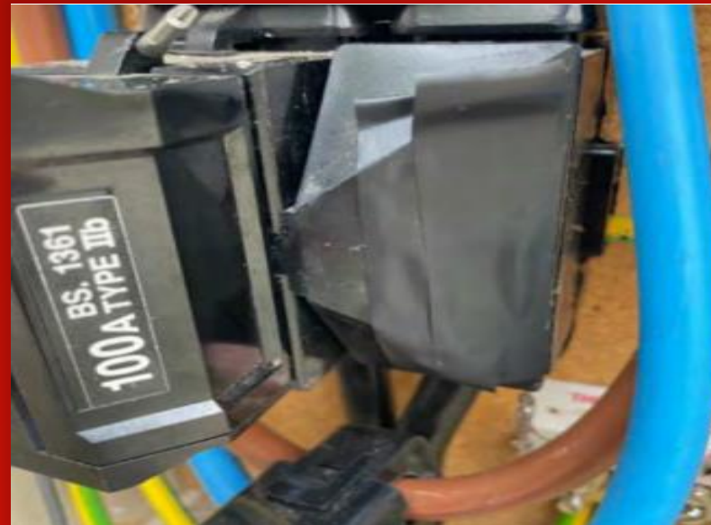
Issues with service head: Damage to service head (ID909)
